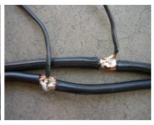
**NB:** Correct preparation of low voltage cable, for end to end soldering. With this low voltage connection technique insulation is not required.
